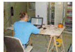
-6- Commissioning of the pulper
