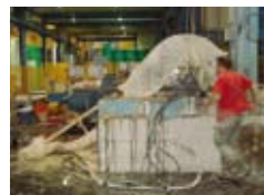
-3- Milling work on drive foundation
